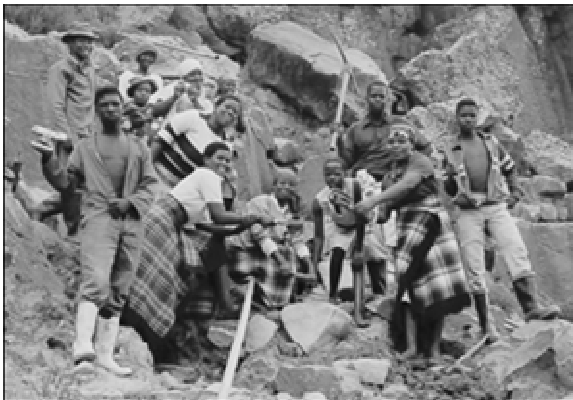
Village team laying a water supply pipe
